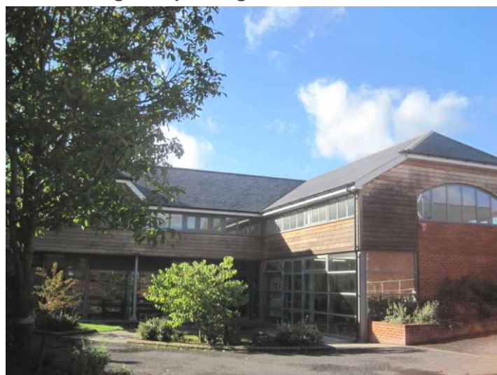
View of Project Workshops
