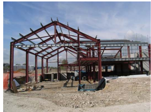
The new Bronze Foundry under construction in April 2009
